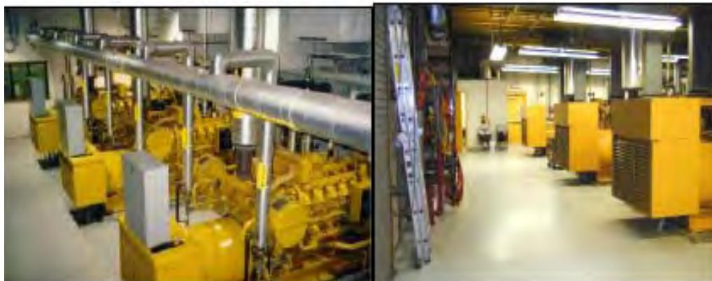
**Figure A-19: Typical Landfill Gas Engine-Generator Sets Installed inside a Building**
