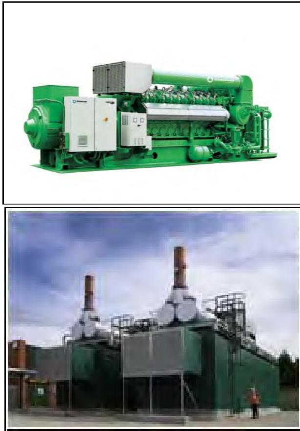
**Figure A-18: Typical Landfill Gas Engine-Generator Set and Pre-Fabricated Enclosures**
