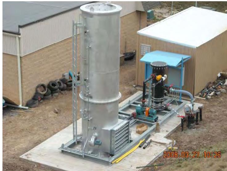
**Figure A-17: Typical Landfill Gas Flare Station**
