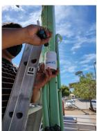
Also, the second CERCA A. C. weather station was installed in the city of La Paz. This station is located in the new CERCA installations; whit this station it is possible to measure precipitation, humidity, temperature, wind direction and speed. Knowing this information allow us to determine how the pollutants found in the air you breathe behave.
