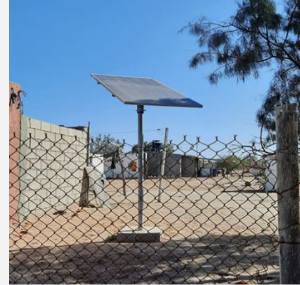
Figure 3 Solar panel of the homes in Puerto Chale 250 [W]
